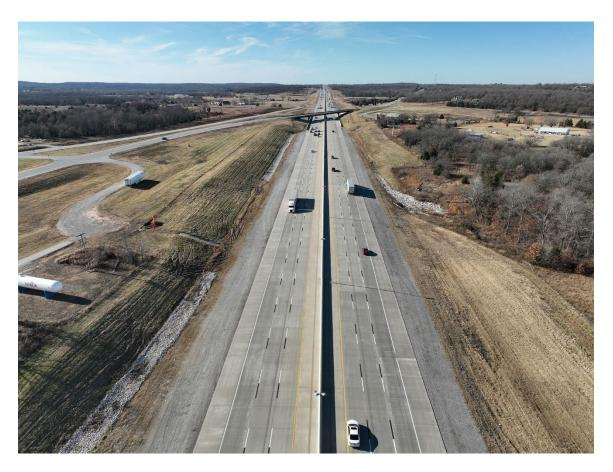
Work will begin by spring 2024 to continue widening the I-44/Turner Turnpike to six lanes from SH-66 (mm 203) to just east of Bristow at mm 197. As shown in the photo, SH-66 crosses above the turnpike and this \$98 million project also will add a new interchange at this location.
